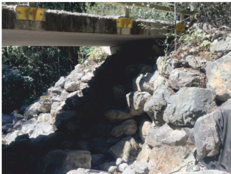
Right Bank Abutment when facing downstream
