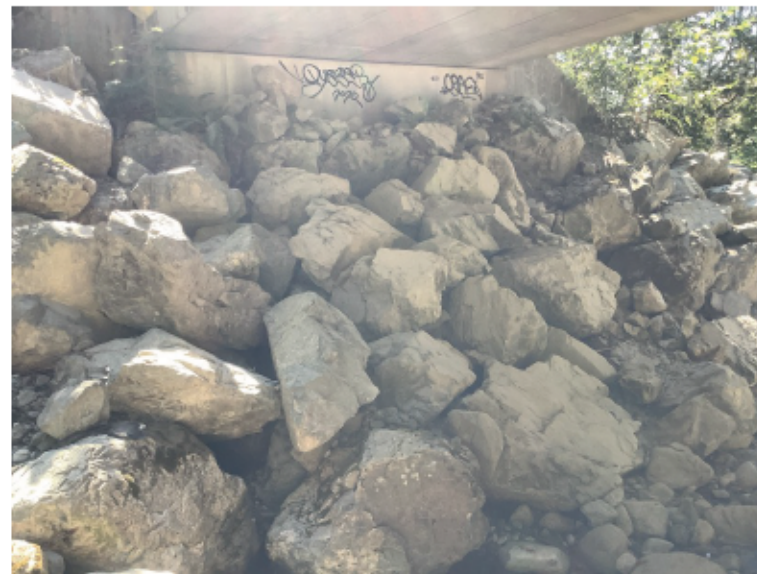
Left Bank Abutment when facing downstream
